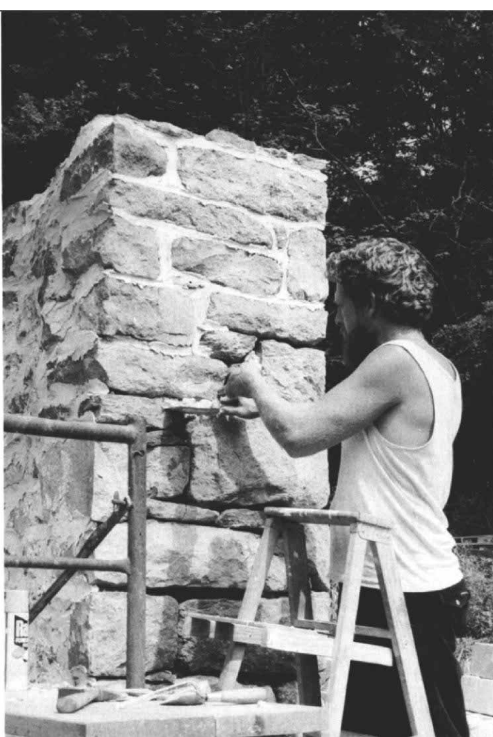
Starting at the top of the wall and working down, Kennedy holds the mortar on a standard mason's trowel (left) and packs the joints with a narrow pointing trowel. After the mortar has set long enough to become crumbly, the joints are dressed (right).
