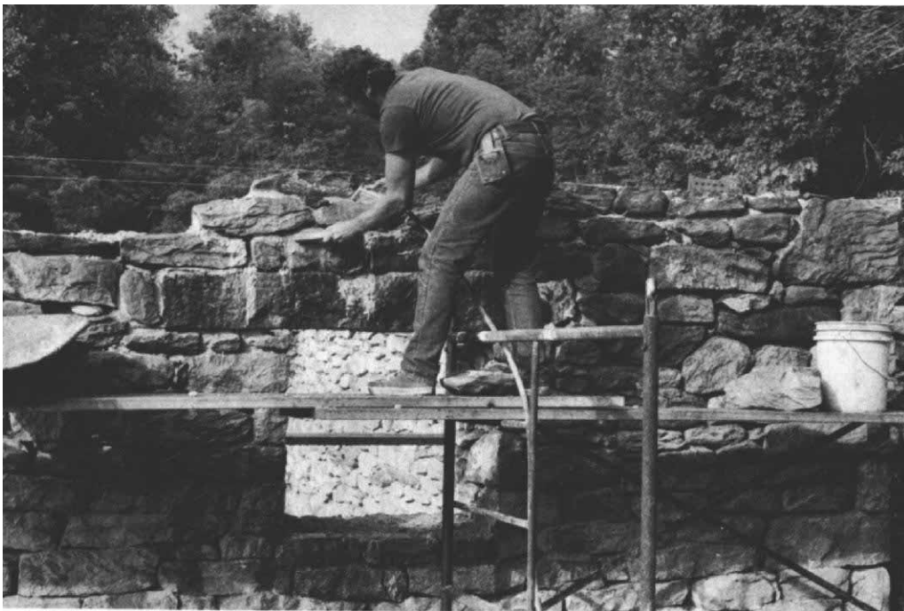
One advantage of bedding the stones first and pointing them later is that you don't need a strong bedding mix. The smears of mortar on the stonework clean up easily with a wire brush and water.
